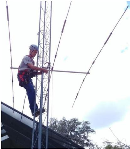
The pole mounted on the Hazer and rotor is about 10 feet so climbing is still needed (15' off the ground) in order to mount the antenna.
