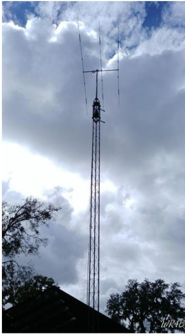
Resurrection of the antenna is complete with the Hazer cranked to the top of the tower.
